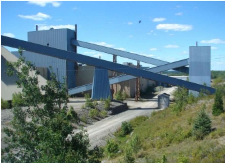
Adex conveyors from administration building
